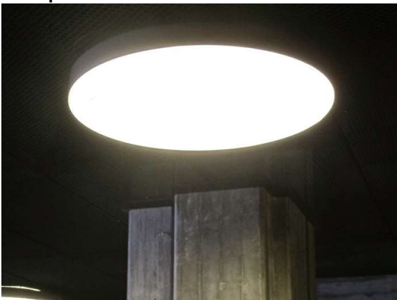
Ceiling mounted Postgaarden, Denmark
